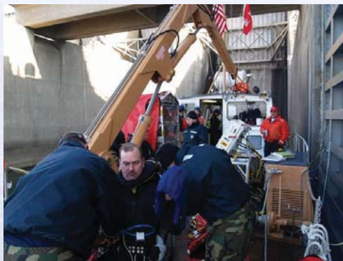
Diver prepares for a dive to measure undermining of the end sill apron on the downstream side of the Dalles Dam located on the Columbia River.
