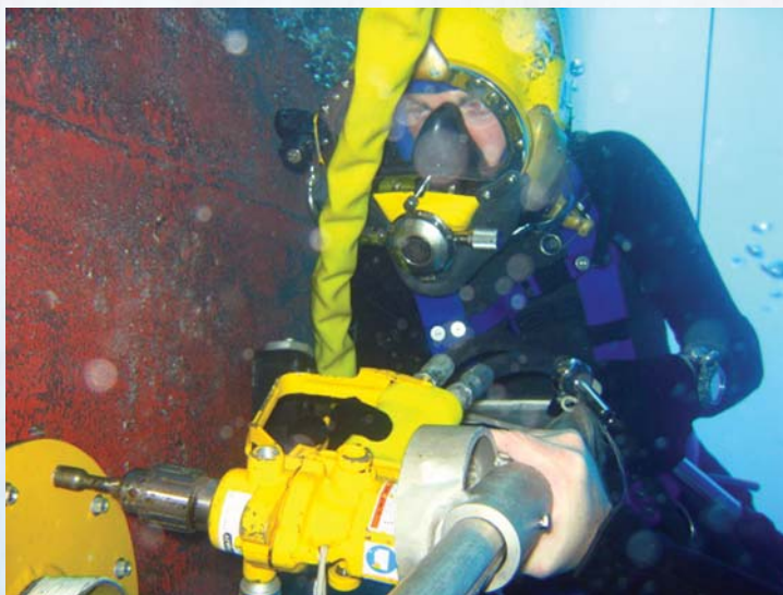
MDSU ONE Det 9 Diver ND2 Gerasimchik installs the hot tap flange.
