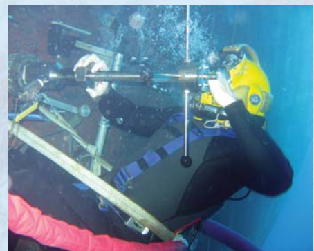
MDSU ONE Det 9 Diver MDV Valentine installs hot tap drill.
