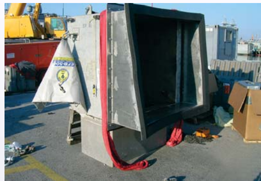
Habitat fabricated and installed to complete dry chamber welding.
