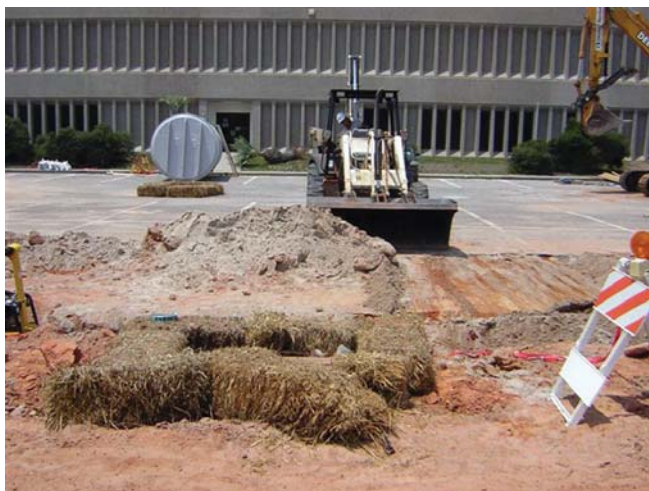
Construction progress, June 2007.
