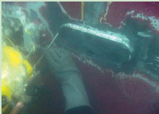
ND1 Justin Pugh Completes cover passes on a doubler plate.
