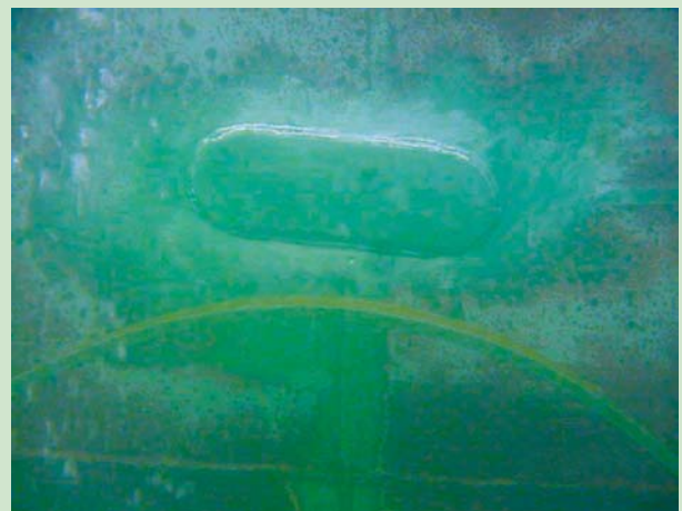
Finished doubler plate wet welded by SWRMC Divers.
