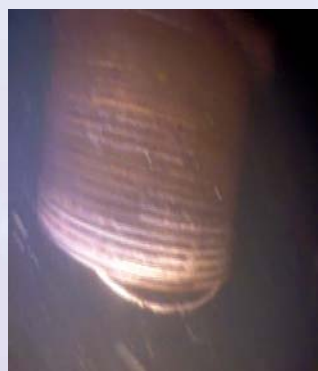
Damaged rudder stock threads.
