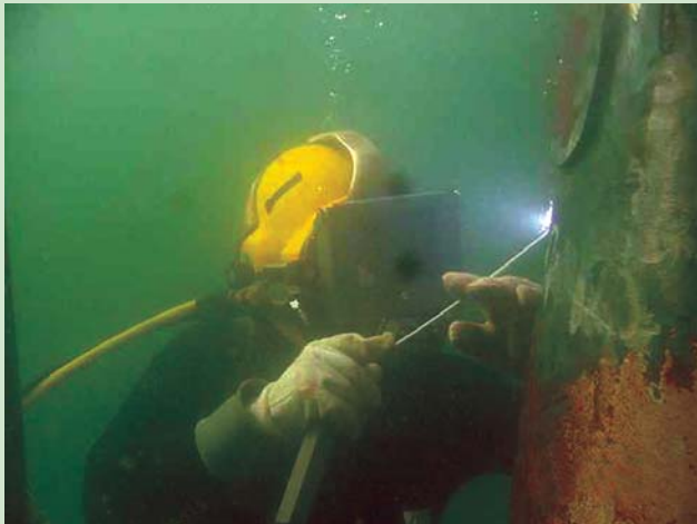
ND1 B.J. Perry wet welds a doubler plate to OGDEN's cracked bow section.
