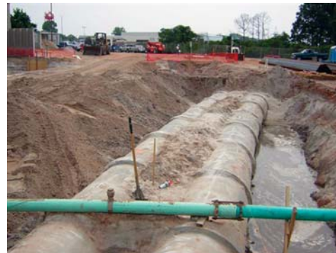
Construction progress, June 2007.
