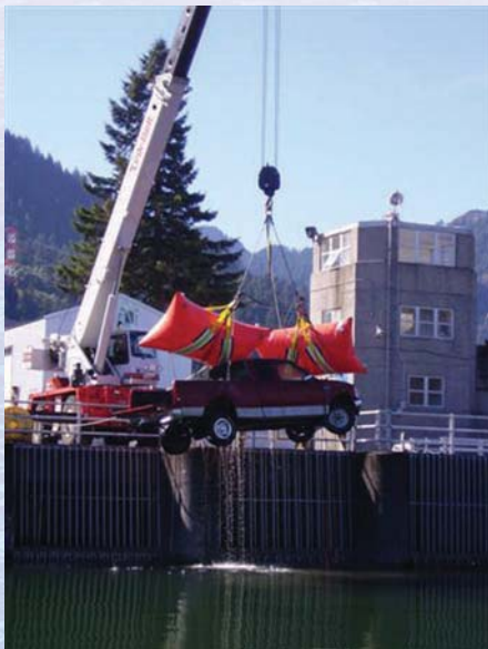
A Ford F-150 is recovered from upstream side of the Bonneville Dam. The truck had inadvertently entered the river creating a potentially catastrophic hazard to several main power units.
