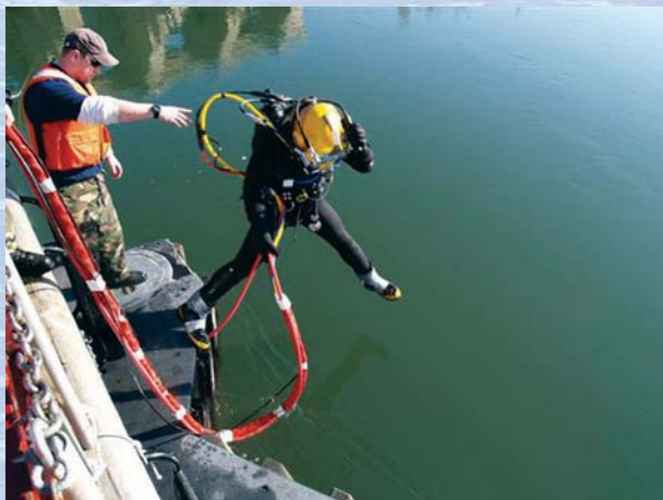
ND1(DSW/SW) Chad Christensen assists NDCS(DSW/SW/SS) Todd Manny entering the water to conduct an end sill apron inspection on the downstream side of The Dalles Dam.
